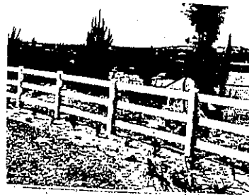
A partial solid bottom is permitted provided the top open portion is at least 35% of the structure with at least 2" openings between the slats.
