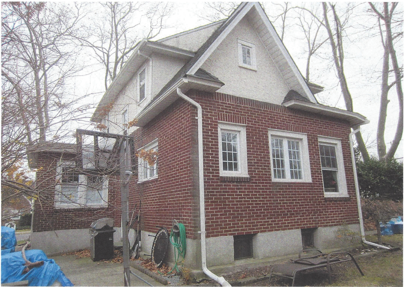
REAR / SIDE ELEVATION NORTH EAST CORNER
