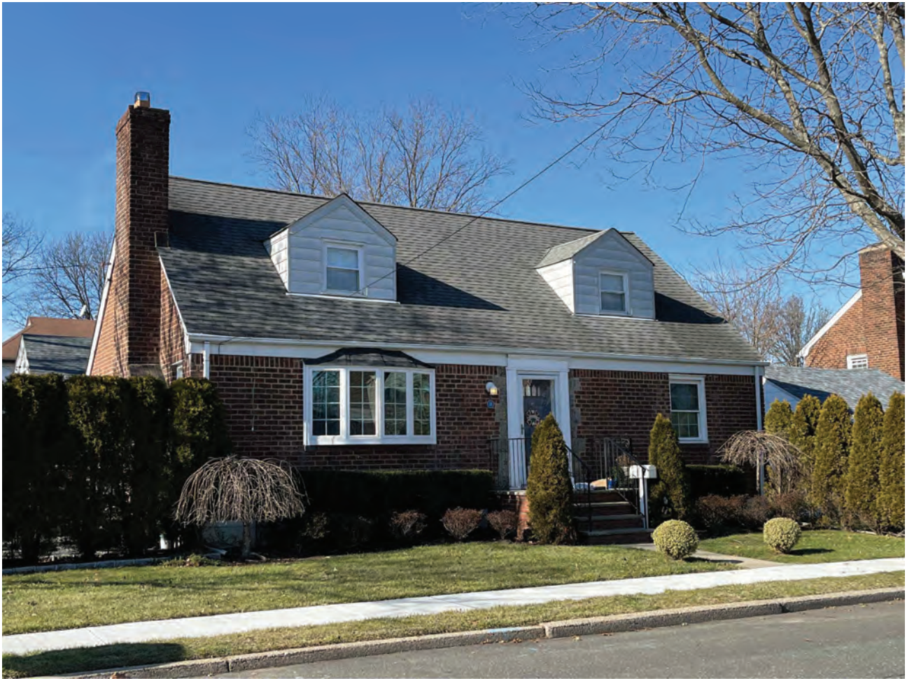
FRONT VIEW (SPRUCE AVE.)
