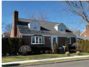
FRONT VIEW (SPRUCE AVE.)
