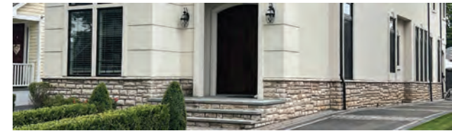
PROPOSED STONE VENEER FACADE ON THE FRONT OF THE HOUSE, BY CAMBRIDGE or EQUAL, COLOR: NATURAL STONES
