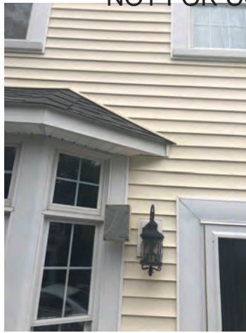
PROPOSED FASCIA, WINDOW & DOOR TRIMS TO MATCH THE MAIN HOUSE, BY "Aztek" or EQUAL, COLOR: WHITE
