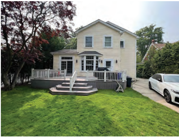
19 HILL St. - REAR VIEW OF HOUSE, ROOF SHINGLES TO MATCH THE MAIN HOUSE, BY "GAF" or EQUAL, COLOR: CHARCOAL
