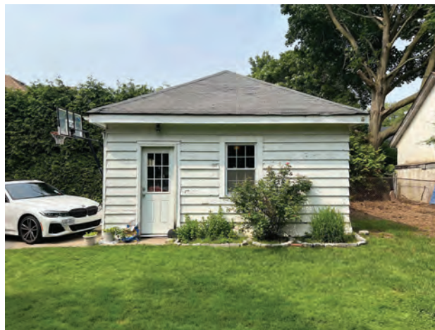
19 Hill St. - South Garage View
