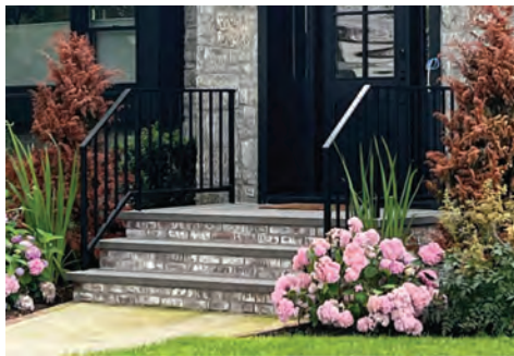
PROPOSED IRON HANDRAIL FOR STEPS, BY "KEY-link" or EQUAL, COLOR: BLACK
