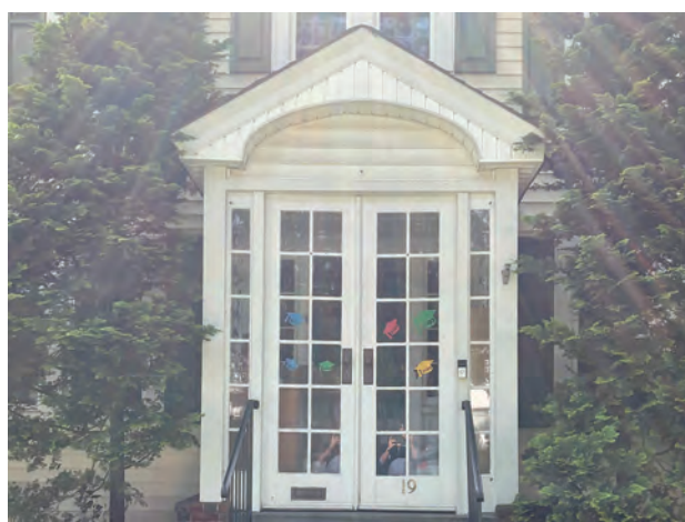
19 Hill St. - Existing Enclosed Vestibule
