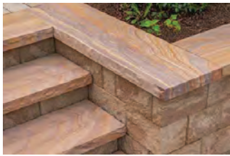
PROPOSED TREAD SLAB FOR FRONT STEPS, BY CAMBRIDGE or EQUAL, COLOR: RAINBOW
