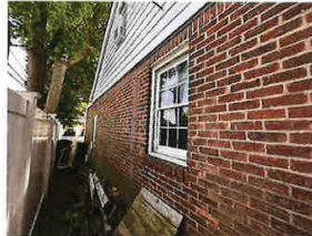
VIEWED FROM BACK OF HOUSE - LOOKING EAST
