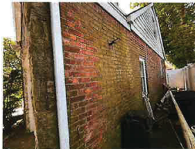
VIEWED FROM FRONT OF HOUSE - LOOKING WEST
