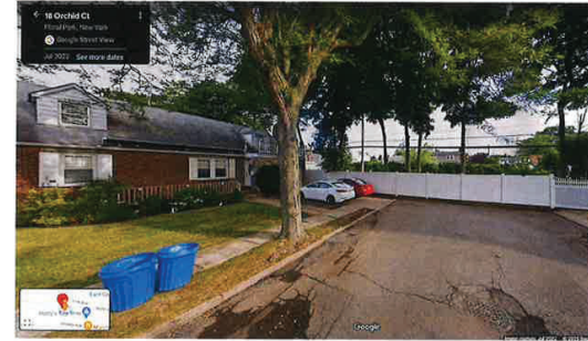
NORTH ADJACENT PROPERTY LONG ISLAND RAILROAD - HEMPSTEAD BRANCH
