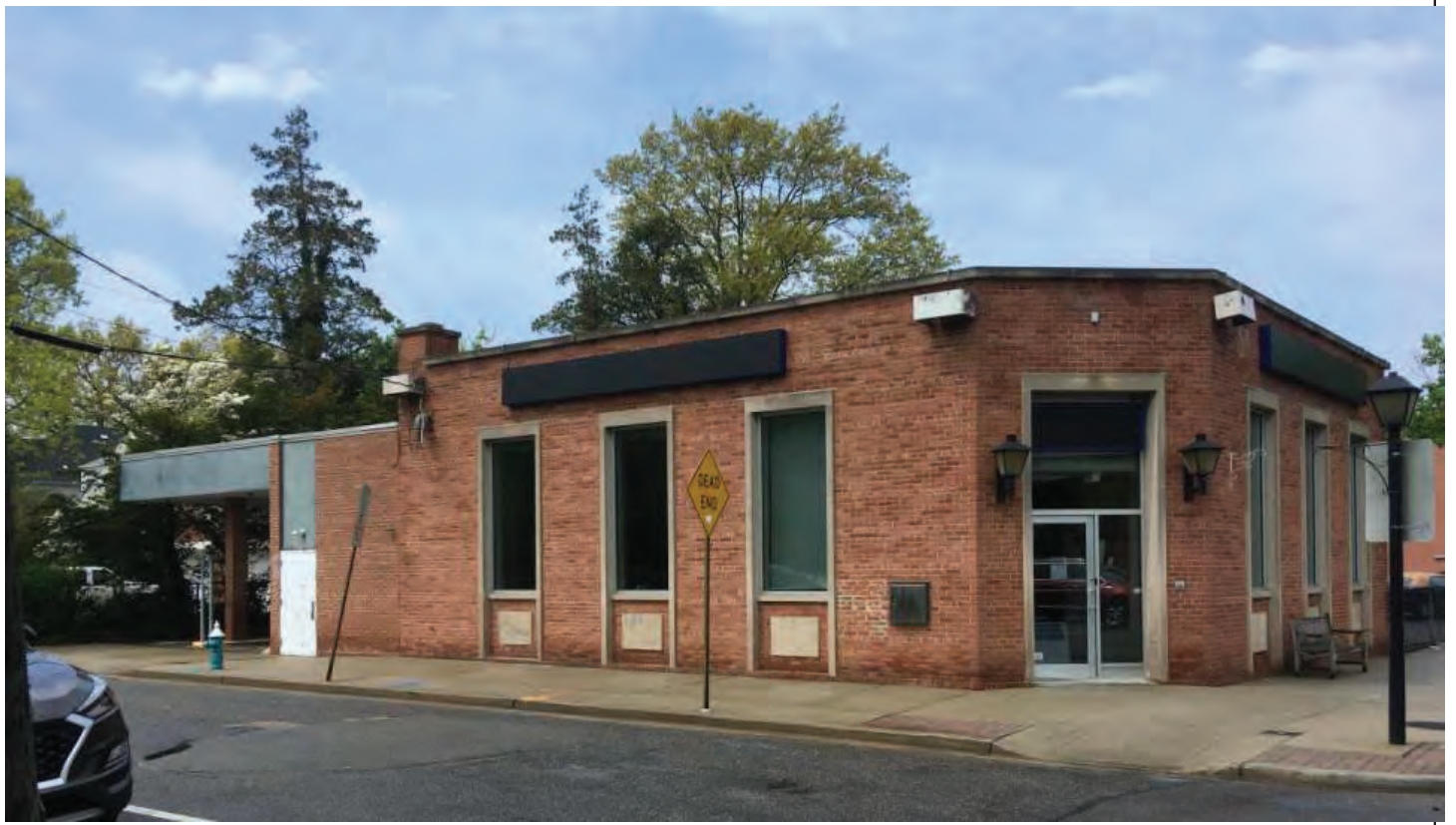
Existing South East corner
