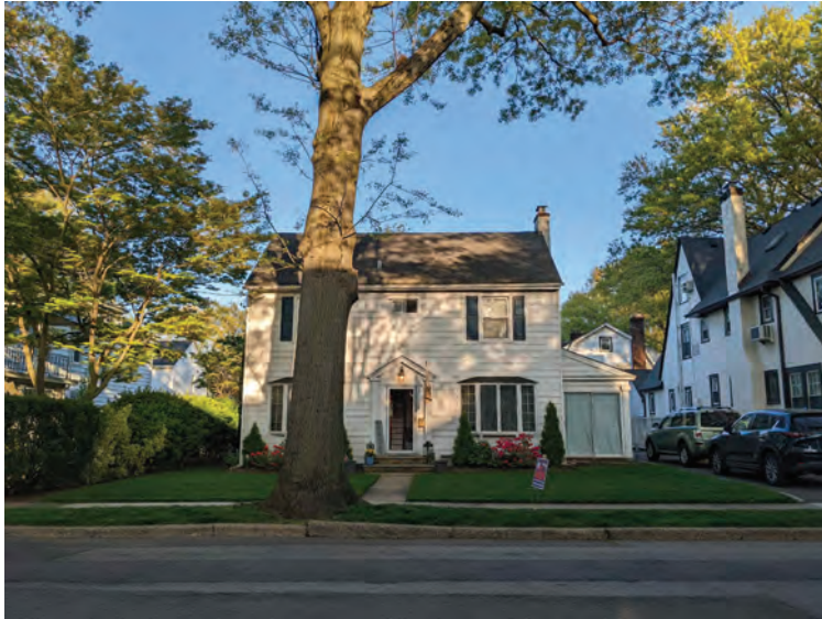
EXISTING PHOTOGRAPH - FRONT (WEST) ELEVATION
