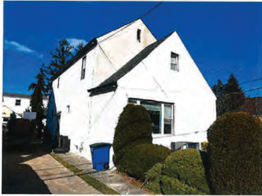
ARRAY LOCATION(S) VIA GROUND
