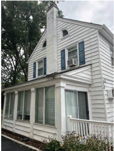
EXISTING PHOTOGRAPH - SIDE (SOUTH) ELEVATION
