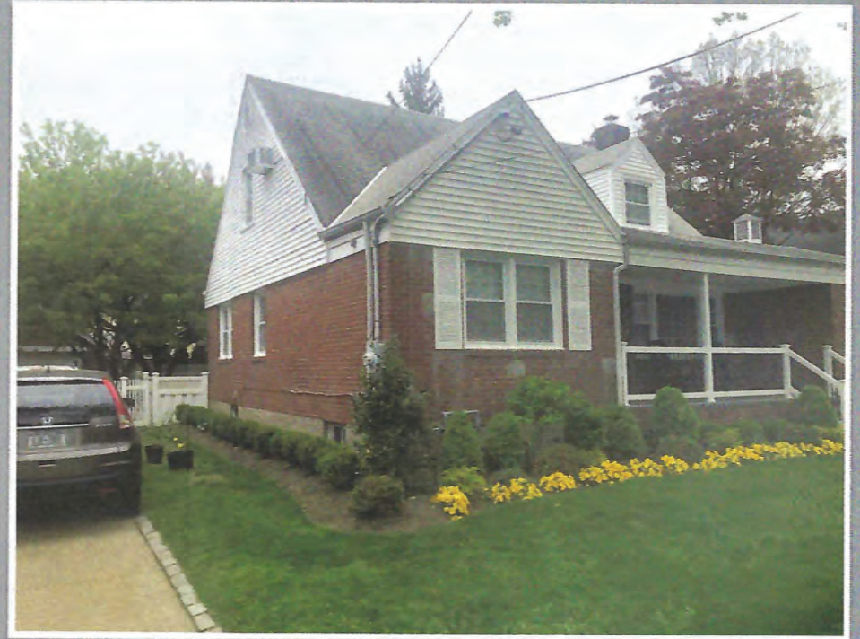
LEFT SIDE FACADE
