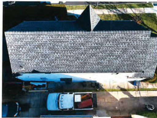
ARRAY LOCATION(S) VIA ROOF
