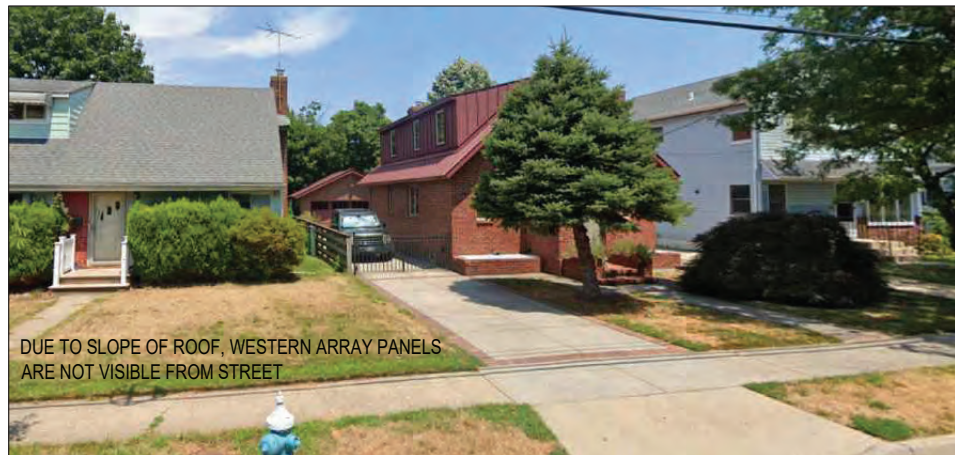
VIEW FROM LEFT SIDE OF HOUSE
