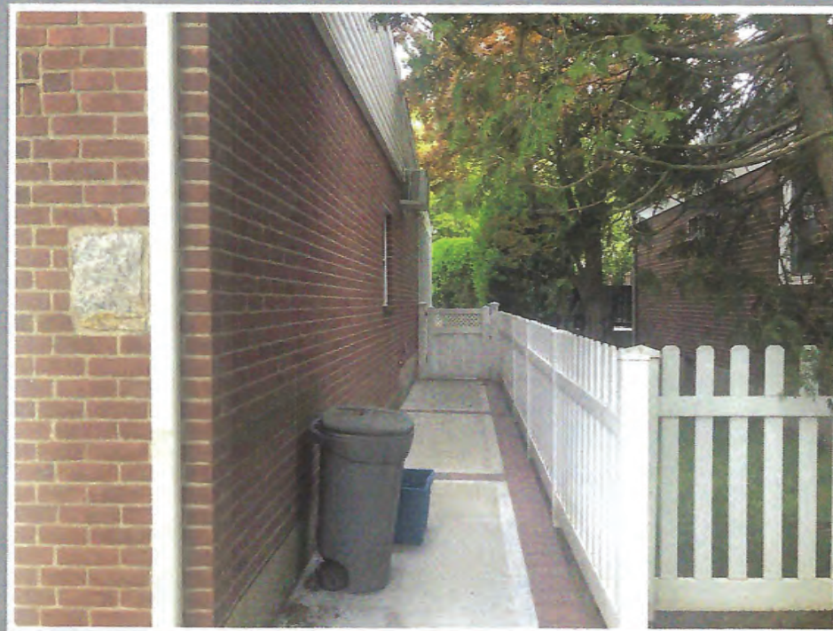
RIGHT SIDE FACADE
