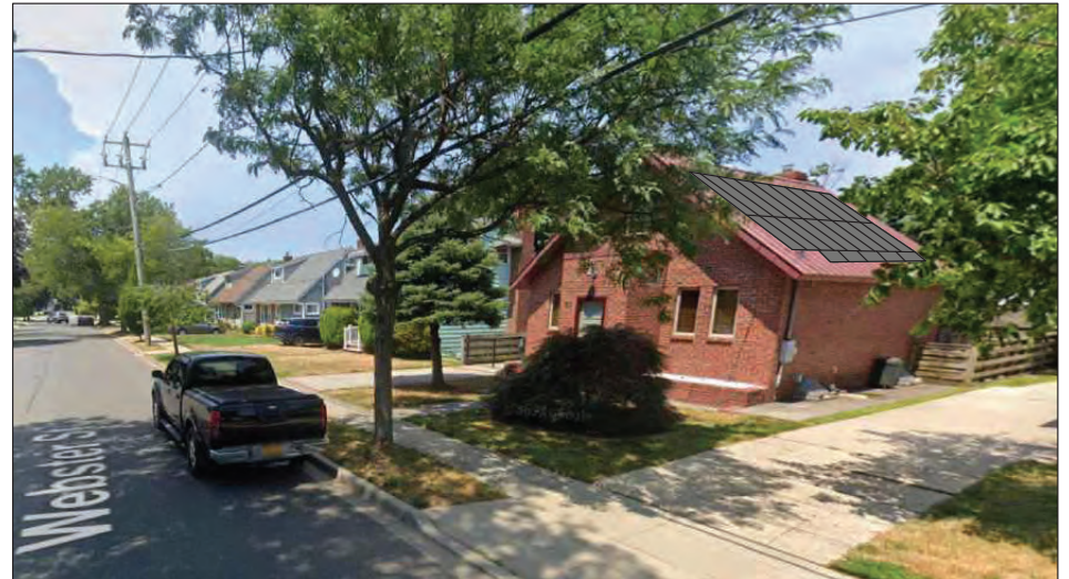
VIEW FROM RIGHT SIDE OF HOUSE EASTERN ARRAY W/ 23 PANELS
