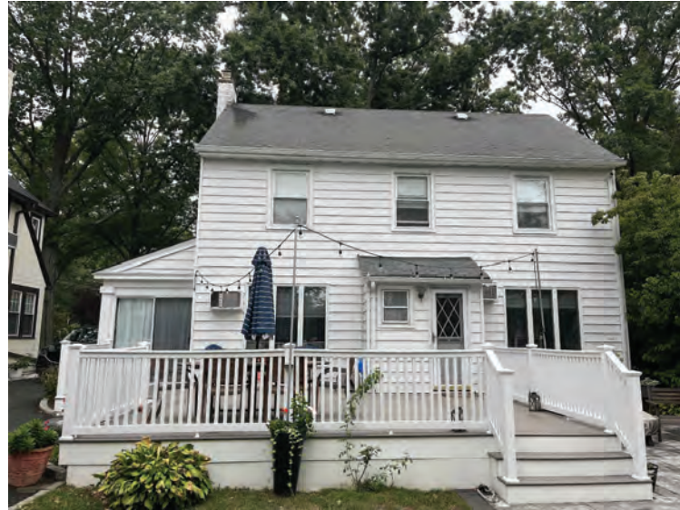
EXISTING PHOTOGRAPH - REAR (EAST) ELEVATION
