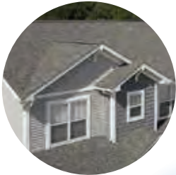
Roofing and Ventilation
