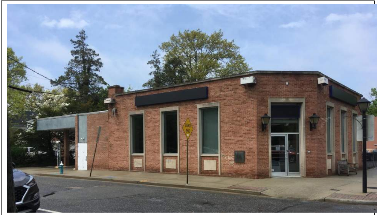
Existing South East corner
