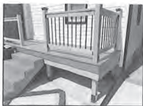
F MAINTAIN: DECK LOOKING SOUTH
