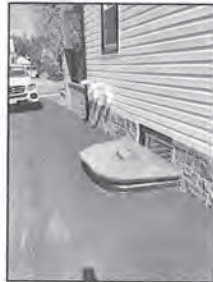
G MAINTAIN: EGRESS WINDOW LOOKING NORTH
