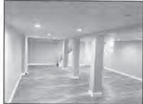
B MAINTAIN: CELLAR LOOKING EAST
