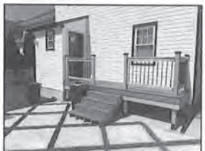
E MAINTAIN: DECK LOOKING NORTH
