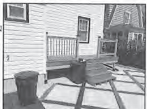
D MAINTAIN: DECK LOOKING NORTH
